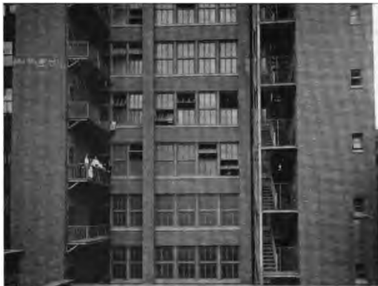
Fig. 2. Two Types of Approved Emergency Exits on one Building.*
